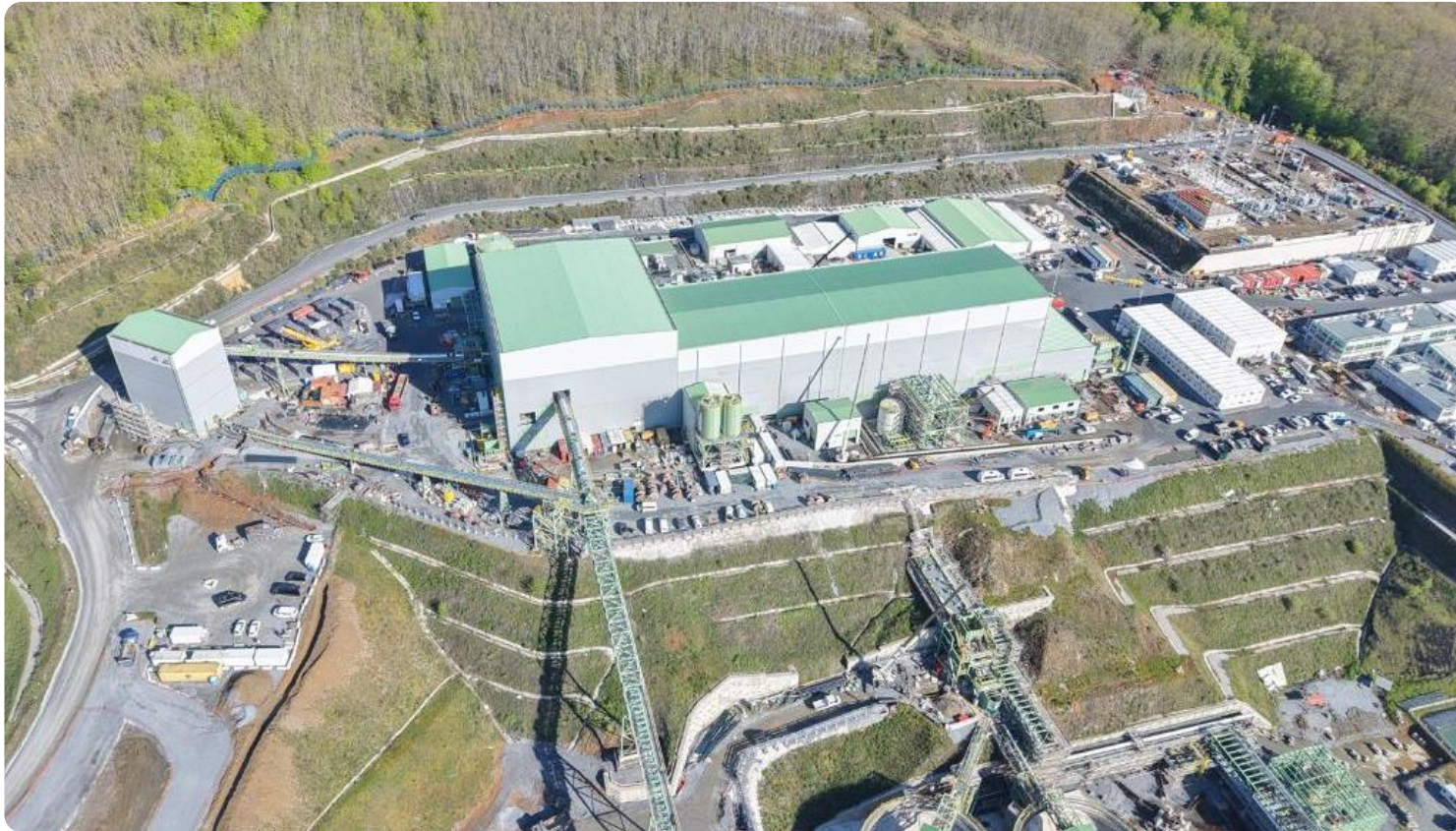
Aerial – process plant
