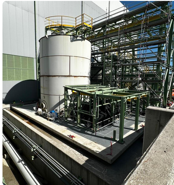
Guar building and tailings pipe rack
