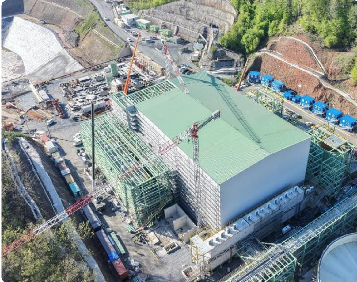
Filtered tailings plant overview, with tank farm progressing shown on the left and the foundation of the compressor building front right
